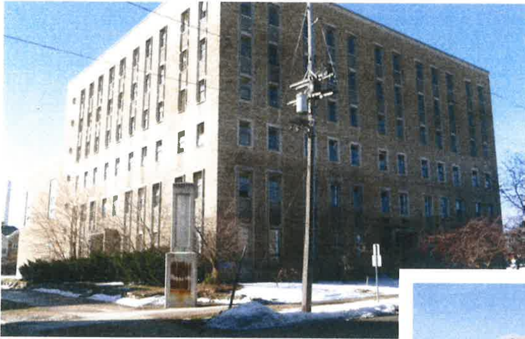
Existing YMCA Before Demolition
